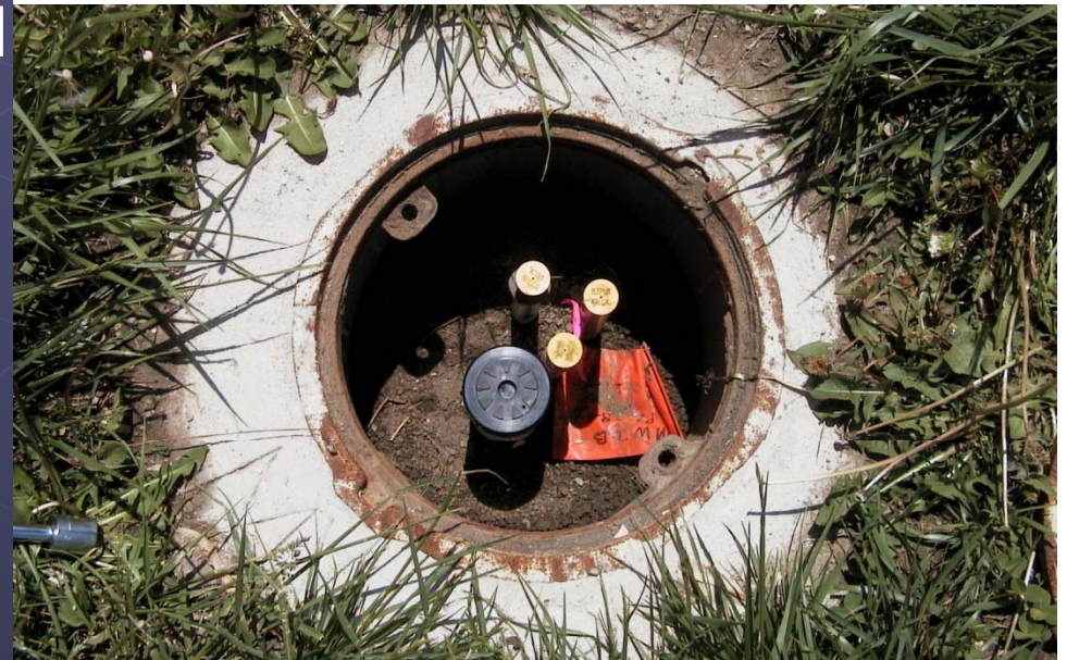
Monitoring Well UE-25 WT#4, Water level about 438 meters (1437 feet) deep Photo by USGS
