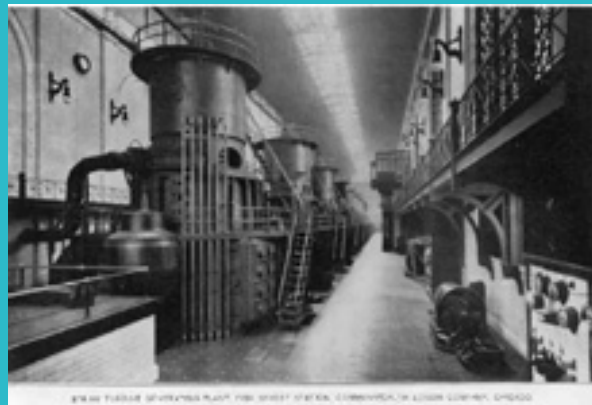
Fiske Street Station steam turbine Chicago, c.1907
