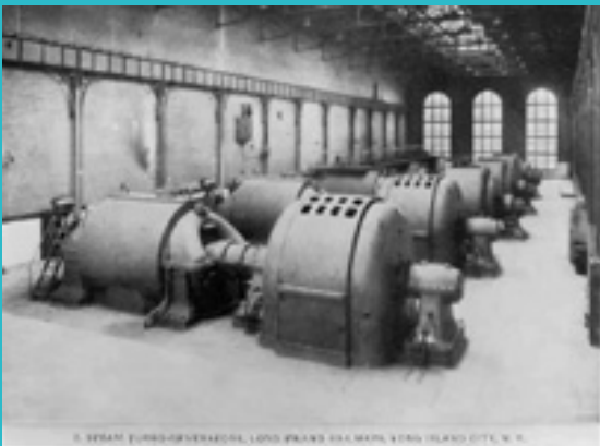
Steam turbo-generators, Long Island railways, c.1907
