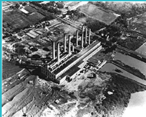
Potomac Electric Power Co. power station near Washington DC, 1939
