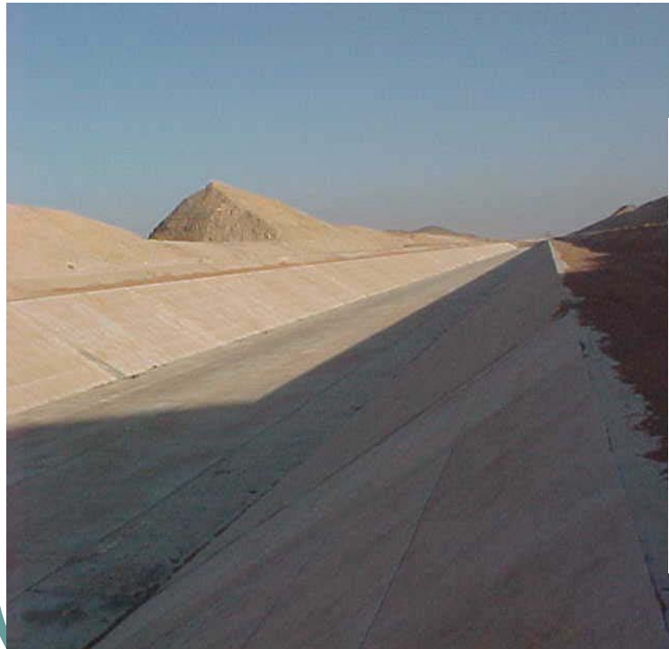
A PART OF FINISHED CANAL
